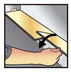
**Step 4.** At the end of the first row, measure the length of the last plank to fit. Be sure to leave expansion spacing at the wall.
